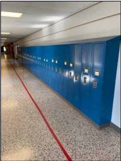
Terrazzo concrete floors are durable and in good condition
