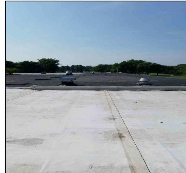
Roof is approximately 5 years old and in good condition
