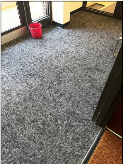
Newer carpet tiles at entrances in good condition
